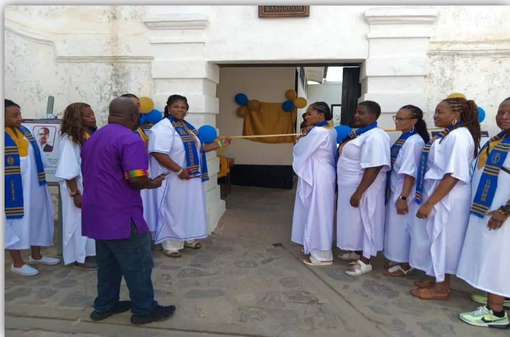
Commissioning Refurbished washrooms at Cape Coast Castle
